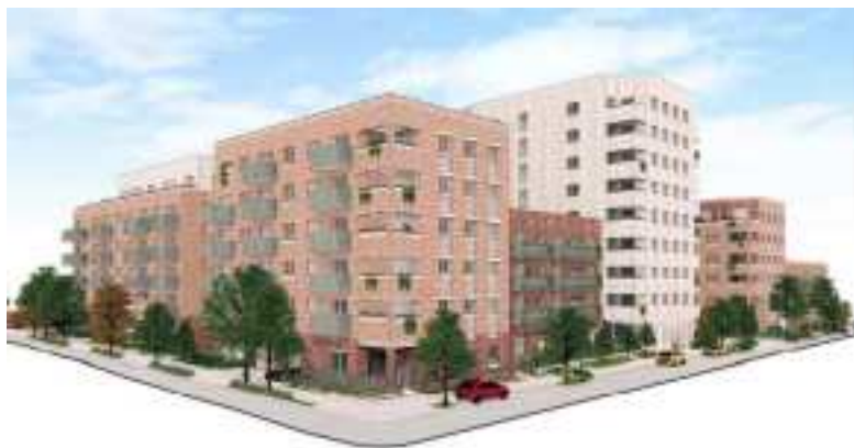
Osborne Road – Plots 9.5 and 9.6/ Eastern view
